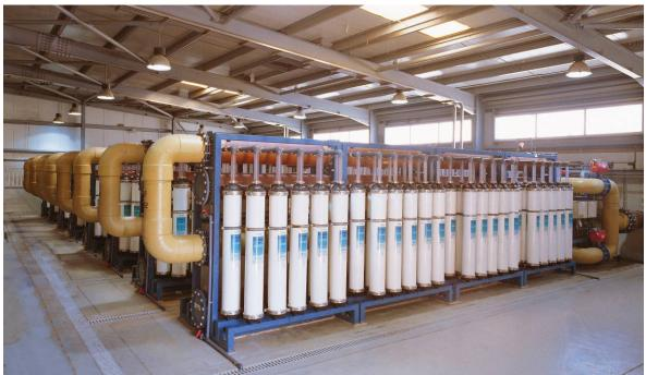
Picture 7: UF Racks - typical configuration Source: KINDASA Water Services, Jeddah
